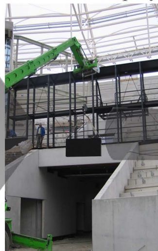
Assemble module by module
