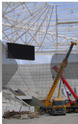
Lift up the screen in position
